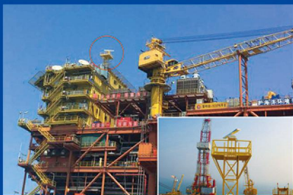
Application in Offshore Oil Platform
